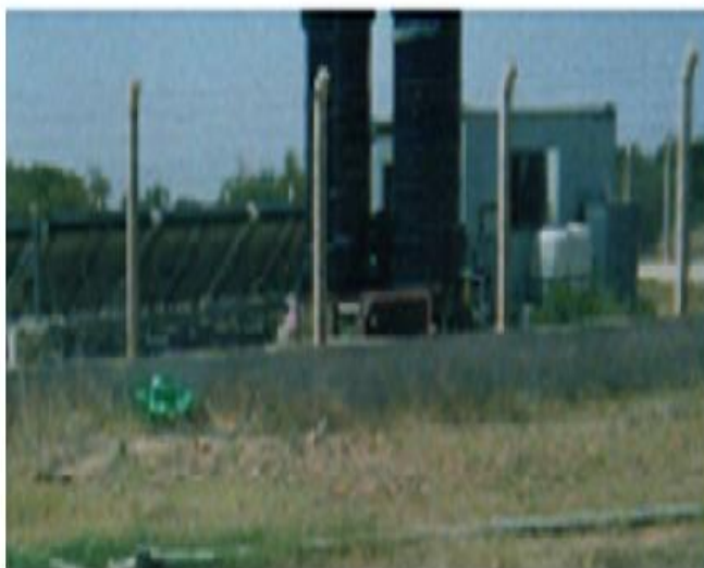
Fig.1. Humidification plant of Hzag
